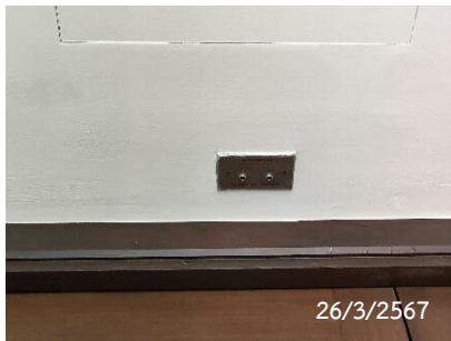
Fire Alarm Indicator Lamp
